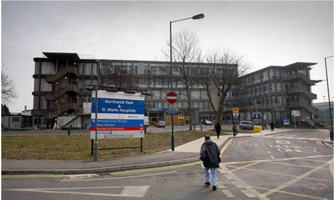
Fig. 2: Northwick Park Hospital. Fachada ingreso principal. John Weeks, arq.
